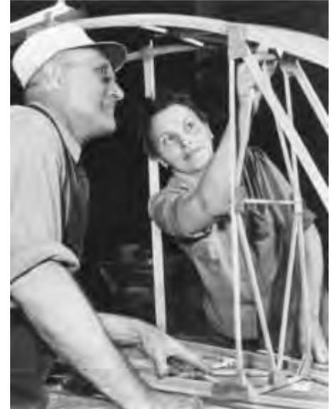
Each joint in a wing of a glider was individually inspected as part of the assembly process at Villaume.
