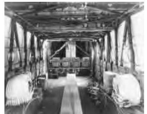
The interior of a CG-13A glider. The design of the welded steel frame, canvas covering on the fuselage, and hinged seats for the glider infantry maximized the available space.
