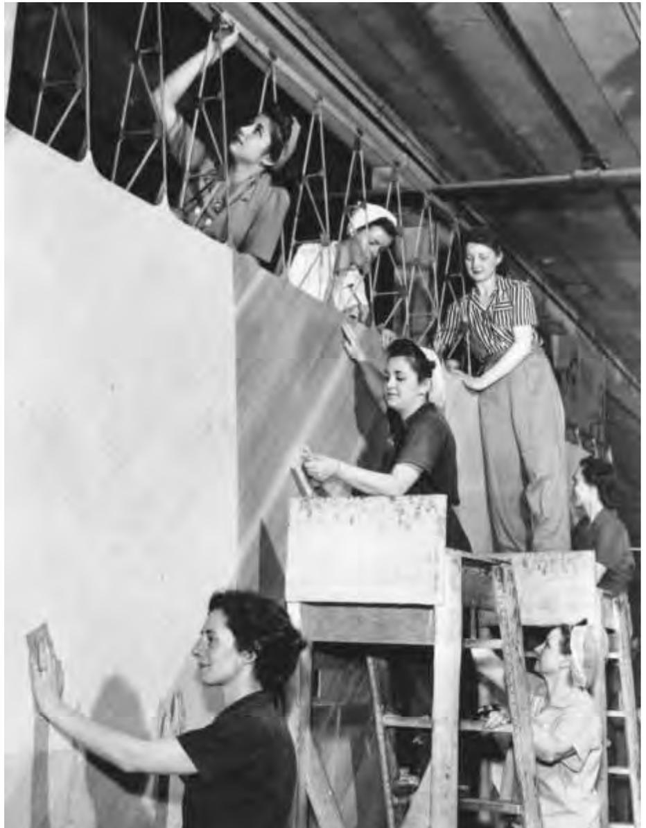
*This photo shows just how much handwork was required to finish the exterior surfaces of a glider wing.*
