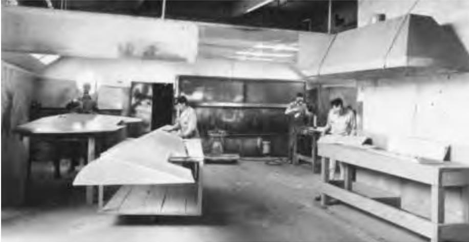
Here workers at Villaume are checking a wing assembly and applying a lacquer with spray guns to a tail assembly (left rear) for a CG-4A.
