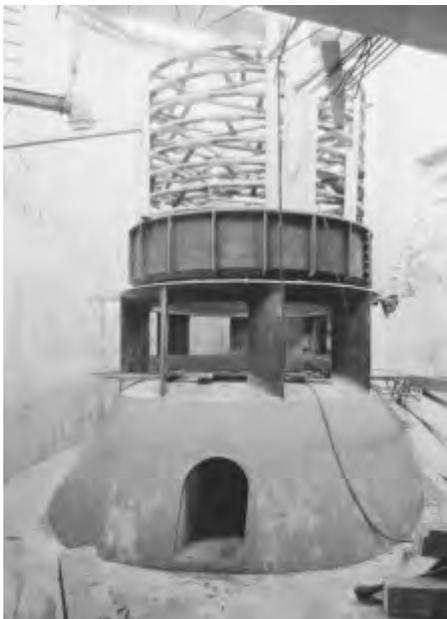
*The hydroelectric plant featured new vertical turbines of the reaction type with a rated power of 4,500 horsepower each. Photo courtesy of the author.*
