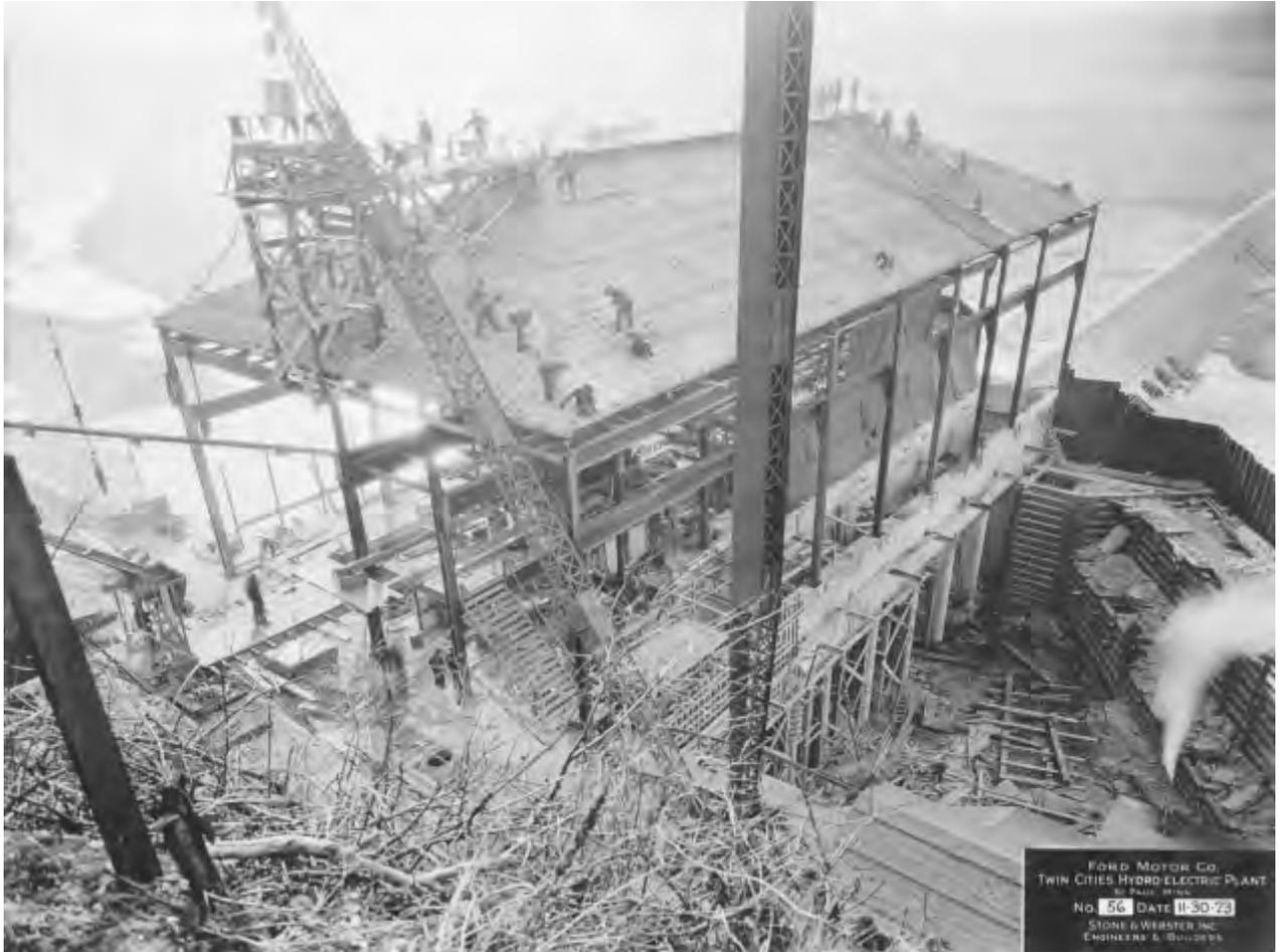
*By November 1923, the structural framework for the new hydroelectric plant was installed. Photograph courtesy of the author.*
