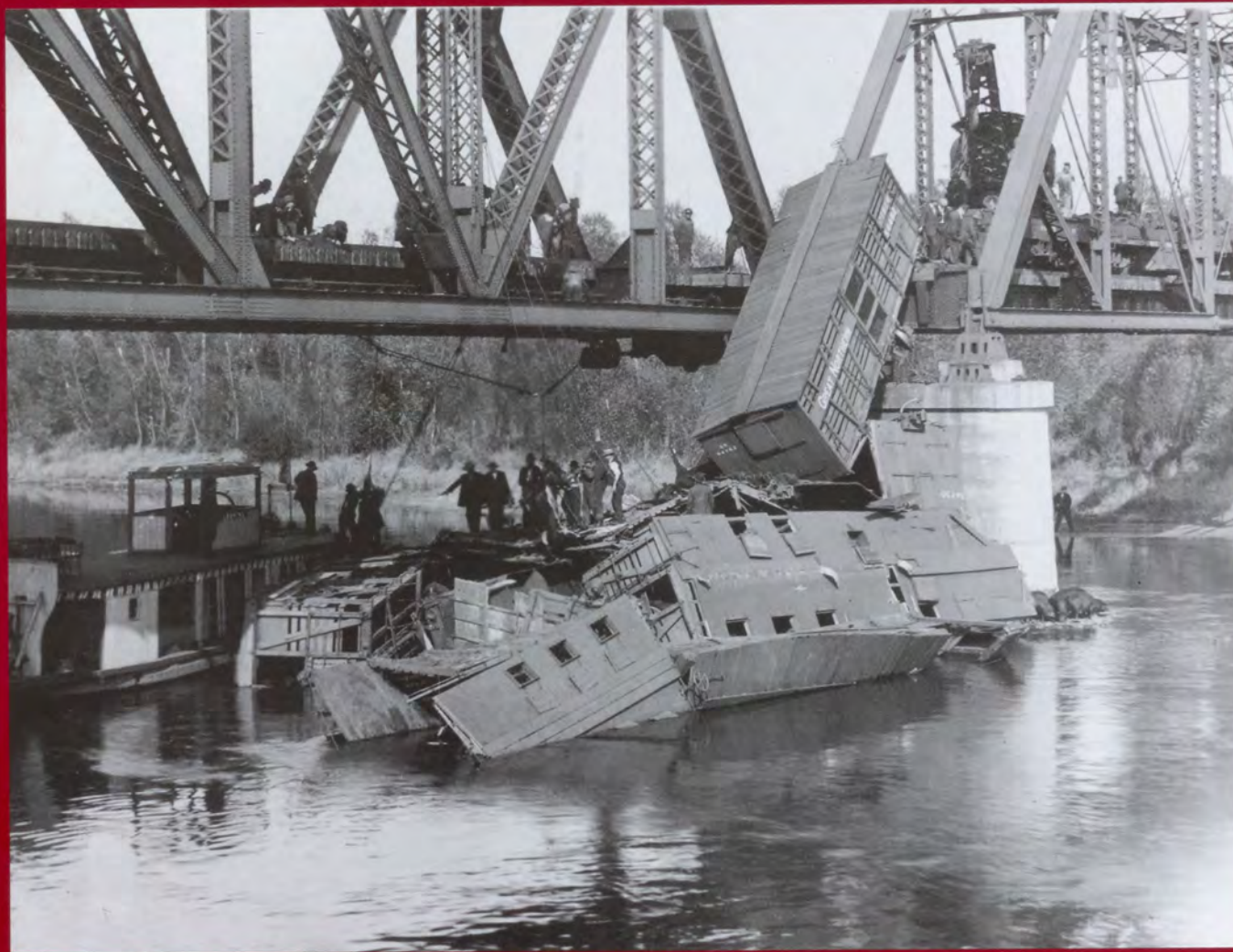
The wreck of Terminal Railway's No. 10 on October 15, 1912 when the 145,000-pound locomotive, tender, and eight cars plunged off the railroad's swing bridge into the Mississippi twenty-five feet below. Photograph from the Davis, Kellogg and Severance Case Files at the Minnesota Historical Society collections. See article beginning on page 4.
