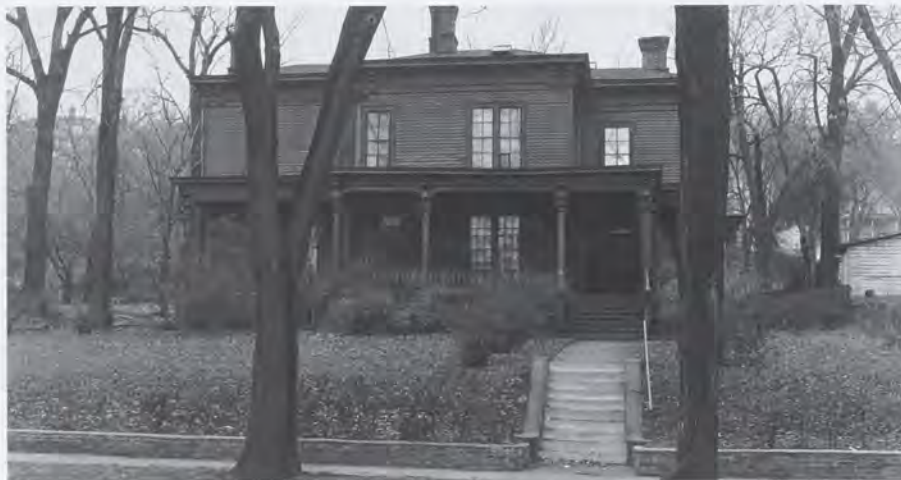
Charles E. Flandrau's house at 385 Pleasant Avenue in St. Paul as it looked in 1942. Minnesota Historical Society photograph.
